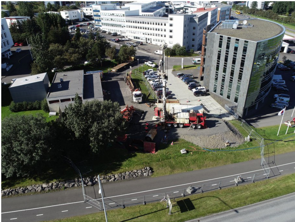
In September 2020, maintenance drilling of one of Veitur's low-temperature geothermal wells began at Bolholt in Reykjavik. The well is one of the most productive ones in the Laugarnes area. It was originally drilled in 1963.
