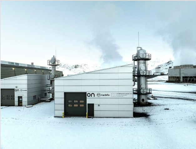
Figure 4. Silverstone capture plant. The plant captures CO 2 and H 2 S from Hellisheiði geothermal powerplants and reinjects it for permanent sequestration.
