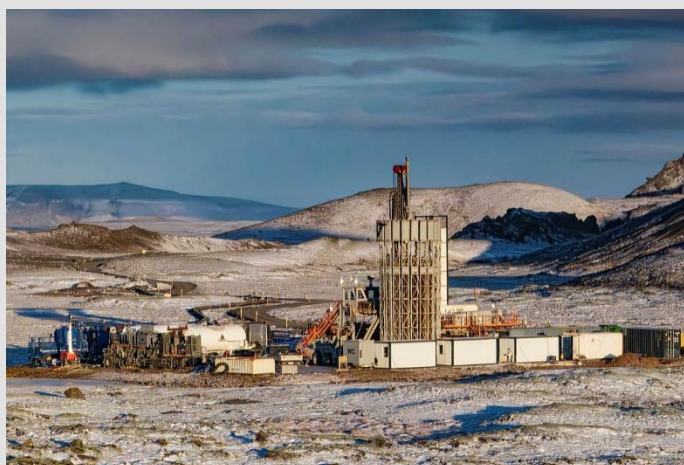
Figure 1. Geothermal research well, HR-02. Drilled in 2025.
